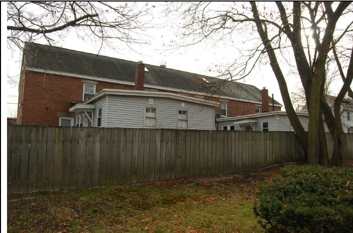
View looking south at rear of 1-7 Gay St.
